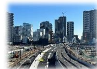
Loop road 2 (between Tsukiji and Shimbashi)
