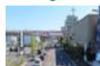
Example of elimination of utility poles
